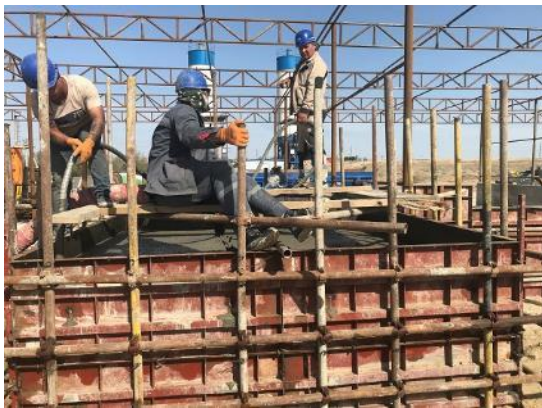
Mock-up for C25/30 Structural Concrete (ABISRP 01)
