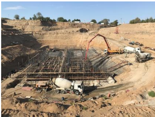
Structural Concrete Works for the Underground Part (Substructure) of the Pump Station Building (ABISRP 01)
