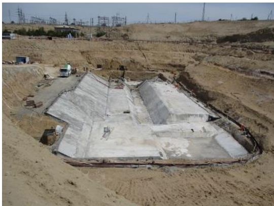
Concrete Bedding (Lean Concrete) and Waterproofing under the Foundation of the Pump Station Building (ABISRP 01)
