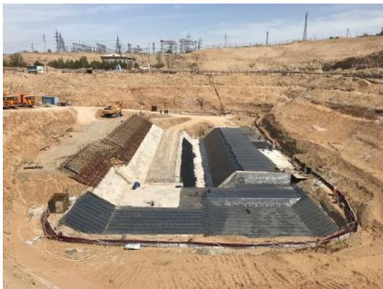
Crushed Stone-Sand Bedding, Concrete Bedding (Lean Concrete) and Waterproofing under the Foundation of the Pump Station Building (ABISRP 01)
