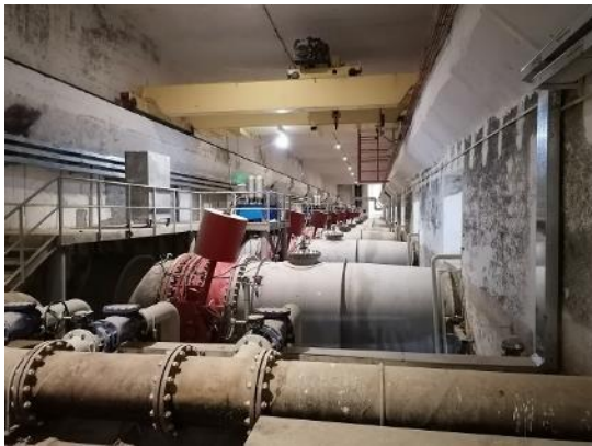
Completion of Replacement of Main Pump Units and Operation of All Pumps in the Current Irrigation Season at Kizil Tapa Pump Station (ABISRP 03 Lot 2)
