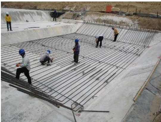
Concrete Bedding (Lean Concrete) and Waterproofing under the Foundation of the Pump Station Building (ABISRP 01)
