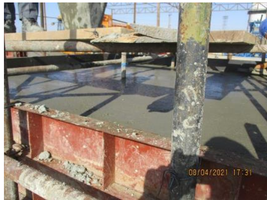
Mock-up for C25/30 Structural Concrete (ABISRP 01)
