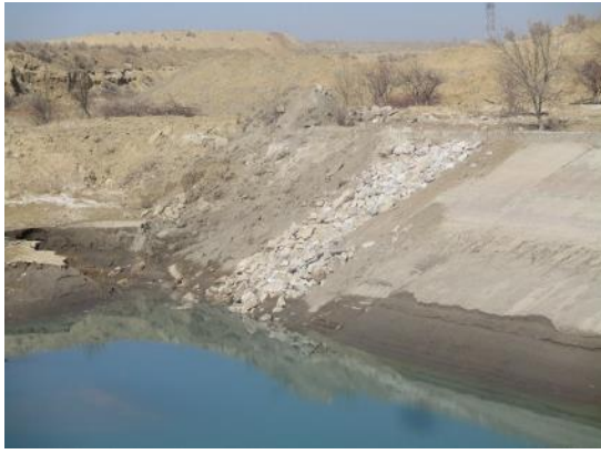
Thickness Check of Existing Metal, Repair of Guide Slots, and Stone Pitching on Regulator ABMK-2 on Hydrosystem Prokop (ABISRP 02)
