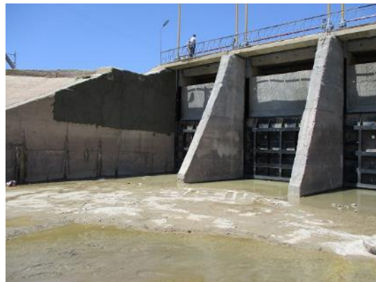
Thickness Check of Existing Metal, Repair of Guide Slots, and Stone Pitching on Regulator ABMK-2 on Hydrosystem Prokop (ABISRP 02)
