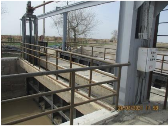
Replacement of Handrails on Hydrosystem Outflow-1 on ABMK-1 (ABISRP 02)
