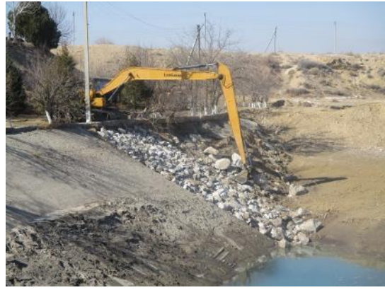
Thickness Check of Existing Metal, Repair of Guide Slots, and Stone Pitching on Regulator ABMK-2 on Hydrosystem Prokop (ABISRP 02)
