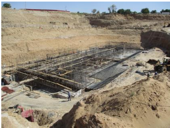
Structural Concrete Works for the Underground Part (Substructure) of the Pump Station Building (ABISRP 01)
