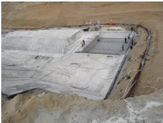
Concrete Bedding (Lean Concrete) and Waterproofing under the Foundation of the Pump Station Building (ABISRP 01)
