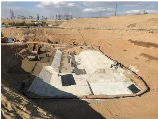
Crushed Stone-Sand Bedding, Concrete Bedding (Lean Concrete) and Waterproofing under the Foundation of the Pump Station Building (ABISRP 01)
