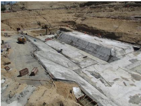
Concrete Bedding (Lean Concrete) and Waterproofing under the Foundation of the Pump Station Building (ABISRP 01)
