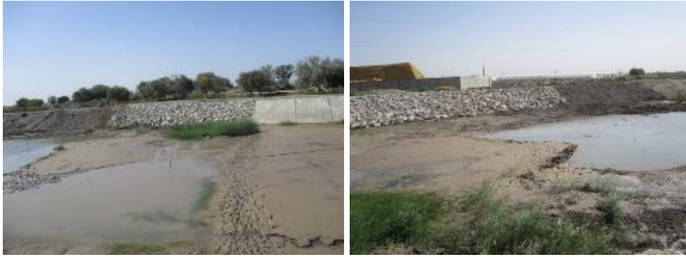
Photos above are from September 2021 Riprap Works at the Downstream of Regulator Verkhnebukharskiy at Hydrosystem Kharkhur (ABISRP 02)
