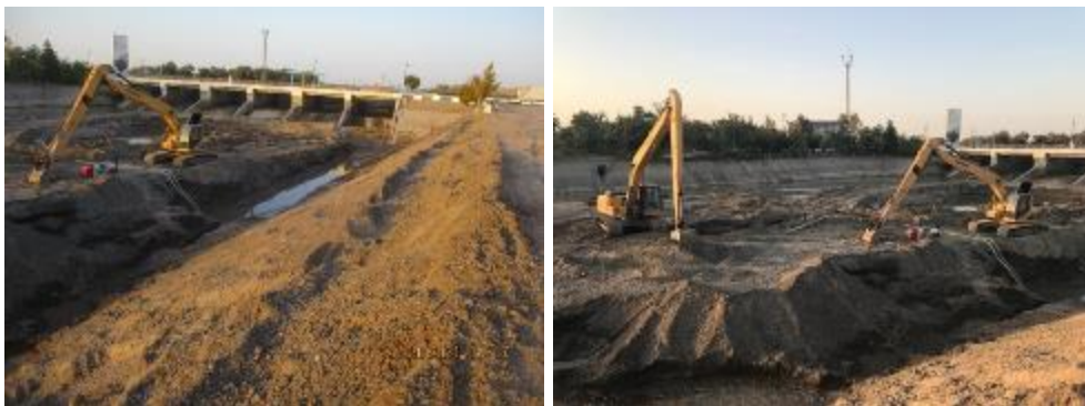
Photos above are from September 2021 Riprap Works at the Downstream of Regulator Verkhnebukharskiy at Hydrosystem Kharkhur (ABISRP 02)
