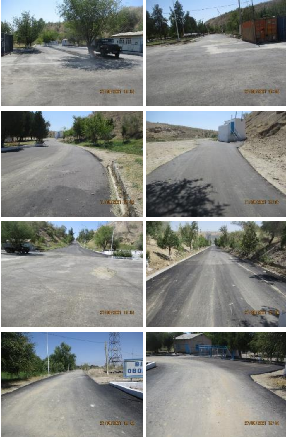
Photos above are from August 2021
