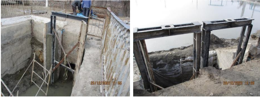
Rehabilitation of Regulating Structures Mayta and Okrabad at Hydrosystem Tashrabad (ABISRP 02)
