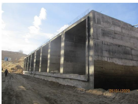
Construction Works of the Trashrack Structure and Transportation Bridge at the Intake of the Pump Station (ABISRP 01)
