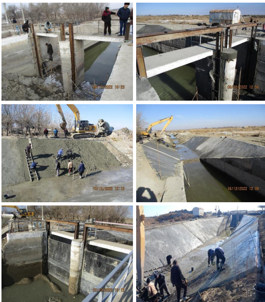
Rehabilitation of Regulating Structure Gijduvan at Hydrosystem Tashrabad (ABISRP 02)
