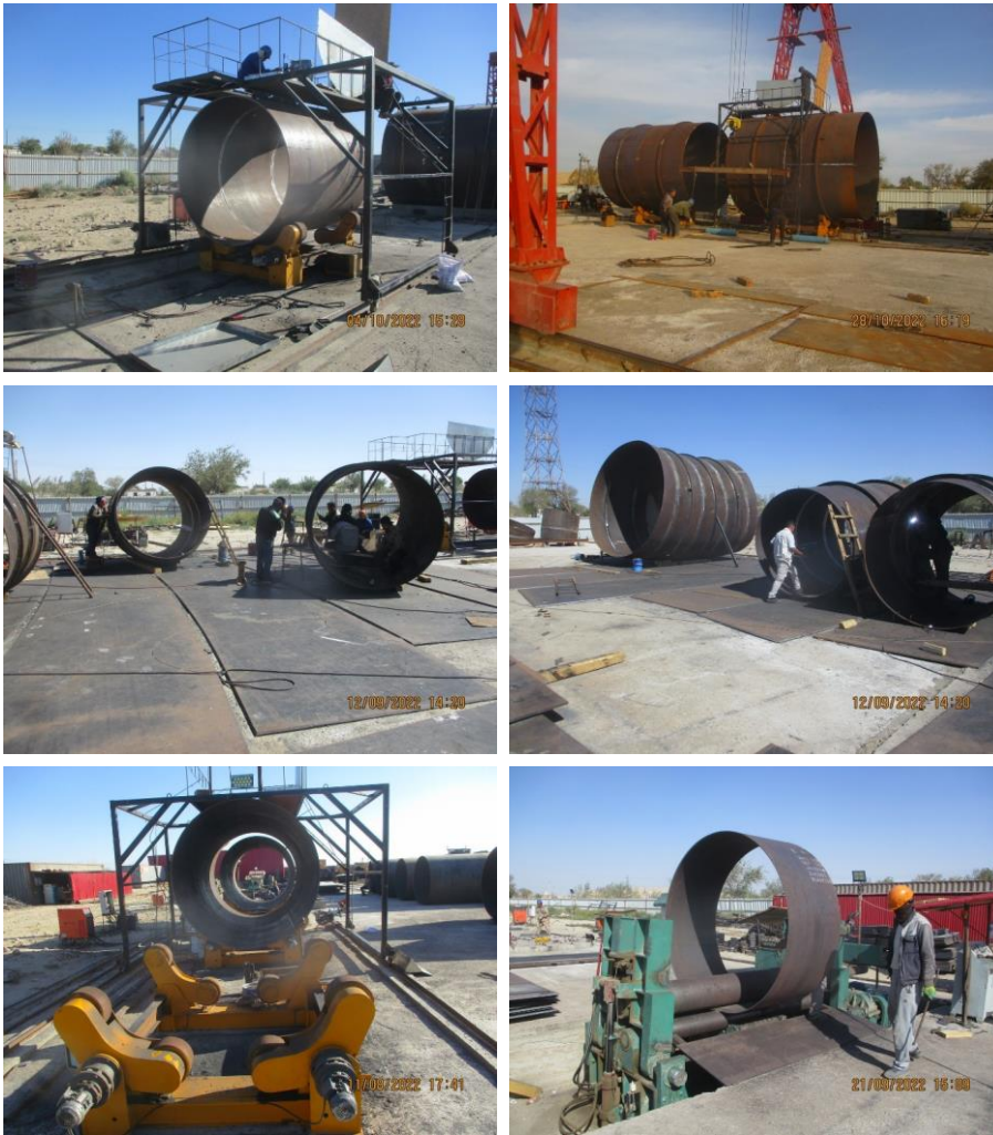
Manufacturing of Discharge Pipes at the Workshop at Site (ABISRP 01)
