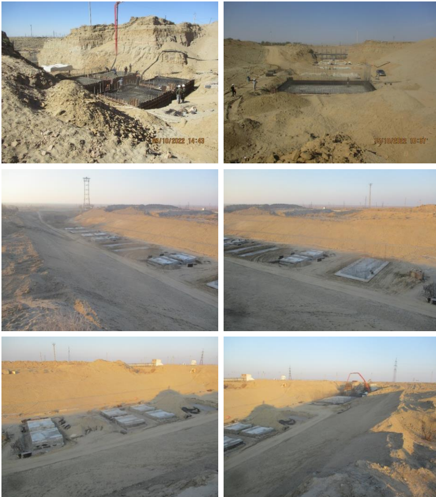
Construction Works of the Intermediate Supports of the Discharge Pipeline (ABISRP 01)
