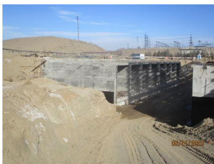
Construction Works of the Trashrack Structure and Transportation Bridge at the Intake of the Pump Station (ABISRP 01)
