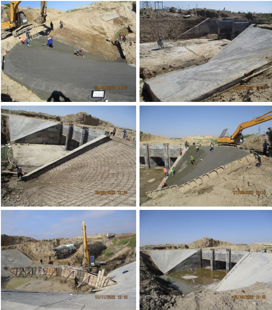
Construction of the Bypass Structure ABK-1 at Hydrosystem Troynik (ABISRP 02)
