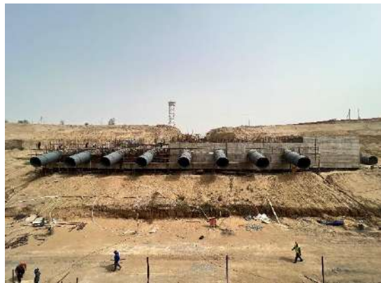
Construction of the Maintenance Butterfly Valve Chamber and Installation of the Maintenance Butterfly Valves and the Discharge Pipeline (ABISRP 01)
