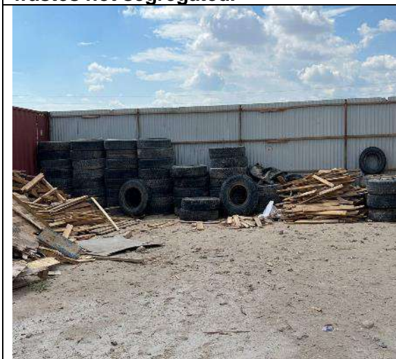
5. Different kind of waste and construction materials not segregated.
