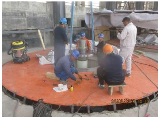
Installation of Main Pump Units (ABISRP 01)
