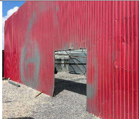
2. Hazardous and flammable material storage area without signs
