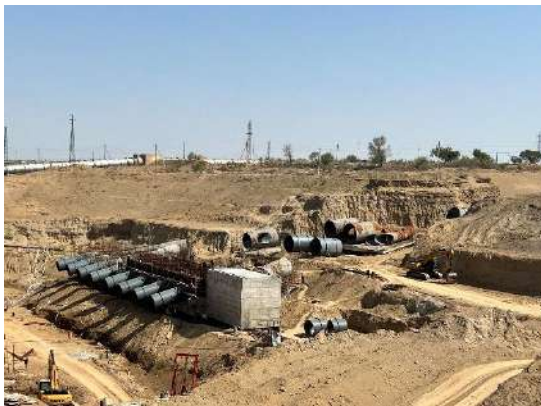
Construction of the Maintenance Butterfly Valve Chamber and Installation of the Maintenance Butterfly Valves and the Discharge Pipeline (ABISRP 01)
