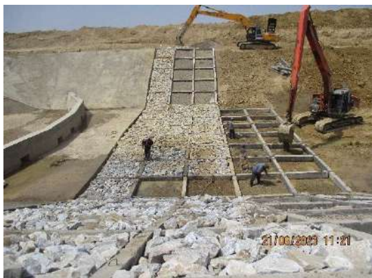
Construction of the Bypass Structure ABK-1 at Hydrosystem Troynik (ABISRP 02)
