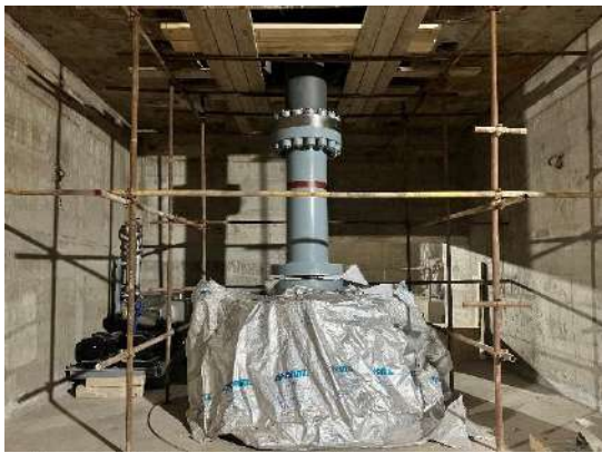
Installation of Main Pump Units #5, 6, 7 and 8 (ABISRP 01)
