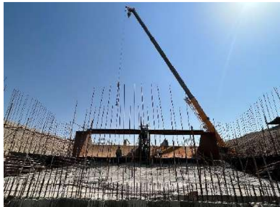
Construction of the Outlet Structure and Installation of the Steel Liner of the Syphon Structure (ABISRP 01)
