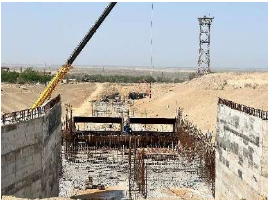
Construction of the Outlet Structure and Installation of the Steel Liner of the Syphon Structure (ABISRP 01)
